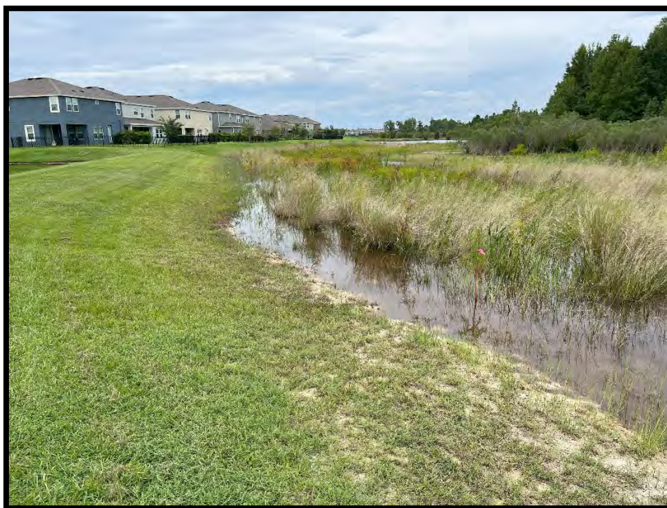
M-38 – Photo point 1, view east
